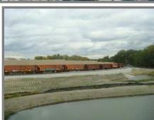
Harbour Contractors, Inc. cut and filled approximately 187,000 CY to provide the proper topography for installation of the southeast connection, loop connection and northeast connection between the IC main lines and the EJ&E main lines.
